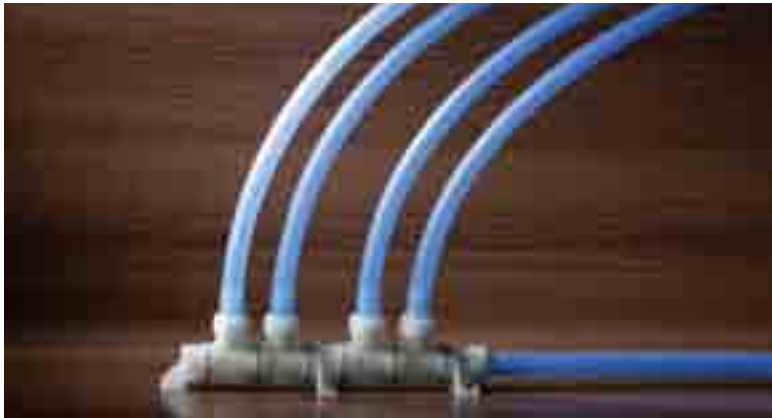
+ The water points are directly supplied with water by the central water distributor
